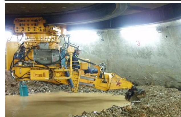
④掘削・沈設
