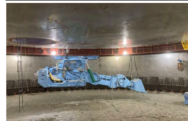
④掘削・沈設
