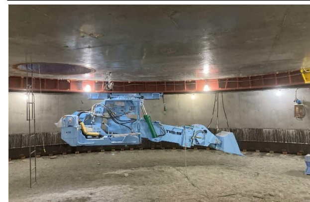
④掘削・沈設
